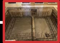
Reinforced Steel Installed to form Pit Walls
