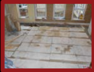
Removal of Concrete Floor Slab
