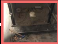
Lift Shaft Build and Lift installed
