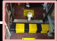
After Pit is Painted
