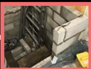
Construction of New Lift Pit Walls
