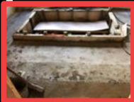
Formwork Installed and Concrete Poured
